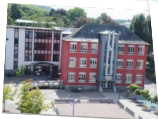
Ecole fondamentale, Ettelbruck, © Christiane Wetzels-Weis
